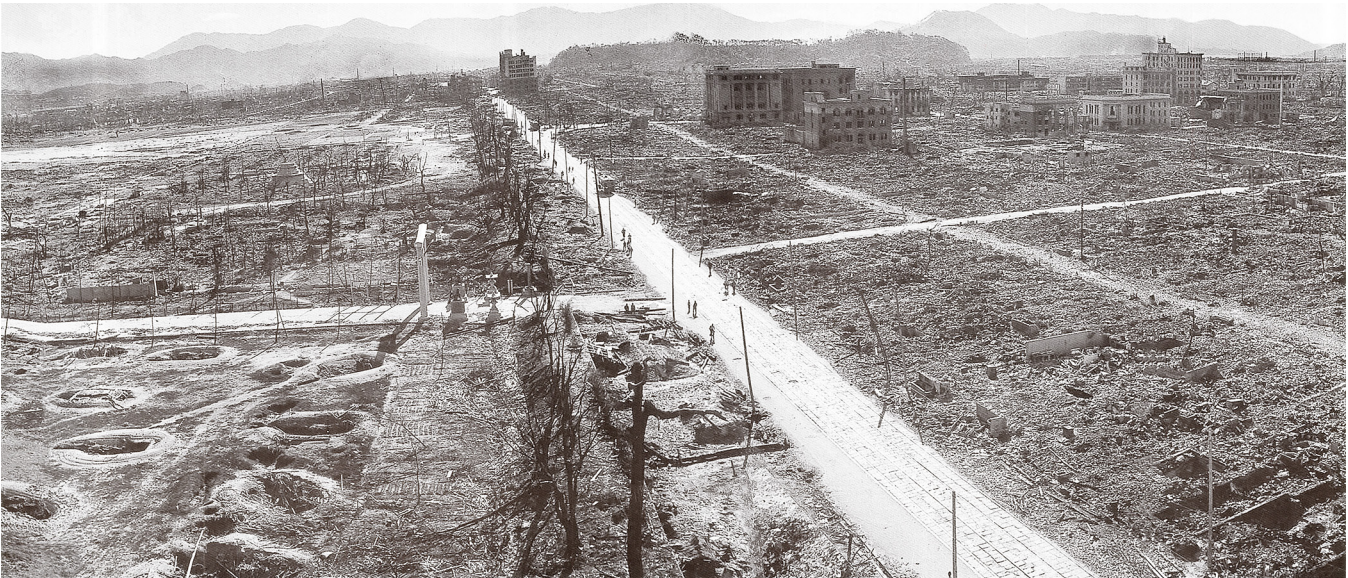
Shigeo Hayashi View from the roof of the Chamber of Commerce Building, 260m north of the hypocenter (Hiroshima), 1945 Photograph Image adapted by Saylor / Morris and Yutaka Sho; Courtesy of the Hiroshima Peace Memorial Museum
